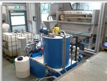
Chemical units are used for preparation and dosing of chemical agents to intensify the wastewater treatment.
